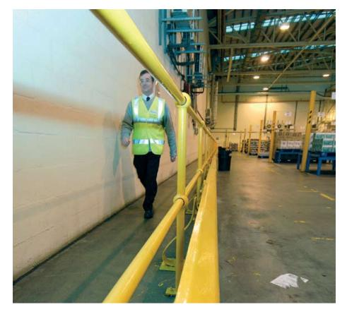
Figure 26 Pedestrian/vehicle segregation
