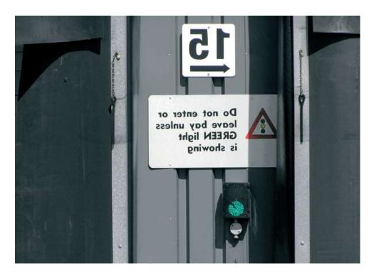
Figure 29(b) The writing on this additional sign has been reversed so it reads correctly when viewed by a driver in their rear-view mirror
