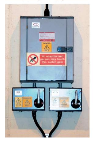
Figure 10 Isolation switch for fixed equipment
