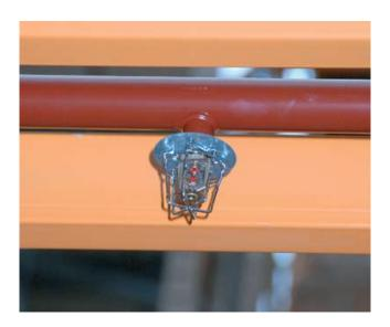
Figures 61 and 62 Parts of a sprinkler system
