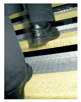
Figure 7 Anti-slip nosing on steps Caution: Standard metal profile can become slippery when wet or contaminated
