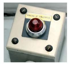
Figure 55 Trapped man alarm
