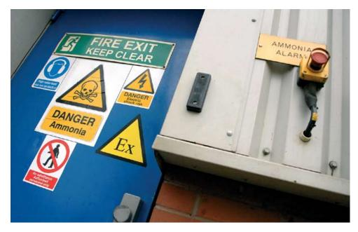
Figure 56 An ammonia plant room emergency exit and alarm
